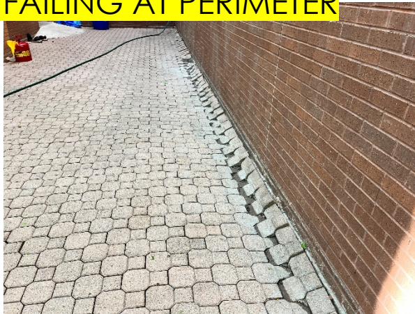
PAVERS FAILING AT PERIMETER
