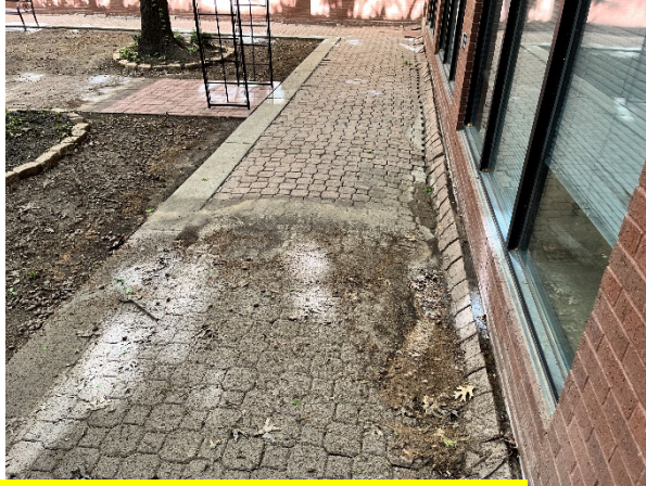
PAVERS FAILING AT PERIMETER
